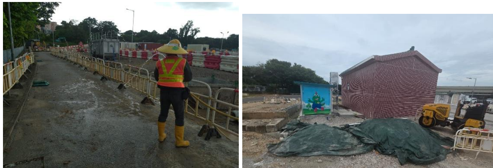
Plate 2.10 Air Quality Mitigation Measures Recorded on site on 16 August 2025
