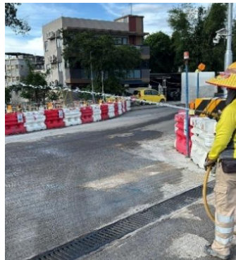
Plate 2.3 Air Quality Mitigation Measures Recorded on site on 8 August 2025
