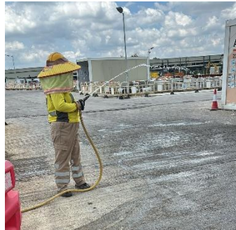
Plate 2.6 Air Quality Mitigation Measures Recorded on site on 12 August 2025
