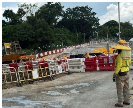
Plate 2.11 Air Quality Mitigation Measures Recorded on site on 18 August 2025
