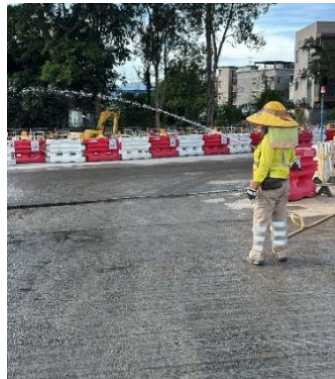
Plate 2.2 Air Quality Mitigation Measures Recorded on site on 7 August 2025
